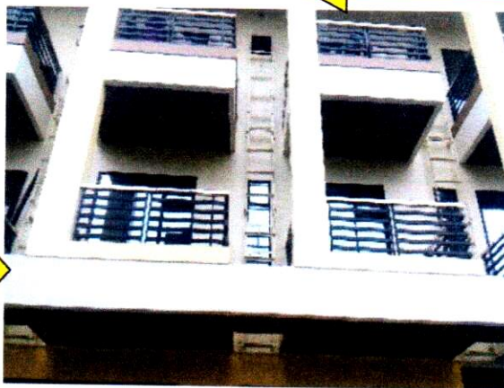
SIDE VIEW OF BUILDING Along Refulgente Alley Road At 2 nd Floor of DC & M Bldg., Room C, D and E
